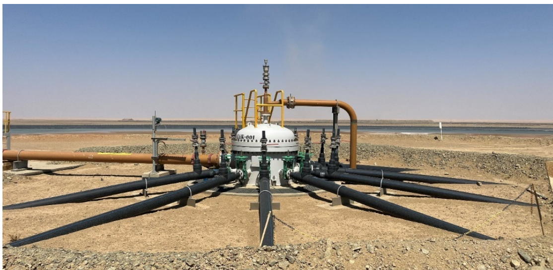
Figure 10 Utilised distribution vessel at Mansourah-Massarrah project
